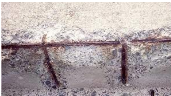
Fig. 5. Exposed reinforcement, absence of protective concrete layer
