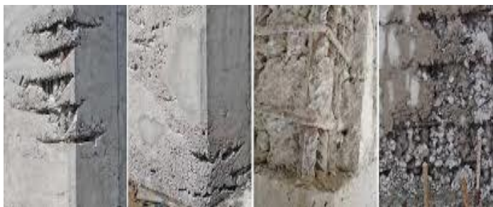
Fig. 6. Voids deeper than the thickness of the concrete protective layer, exposed reinforcement, debris in concrete
