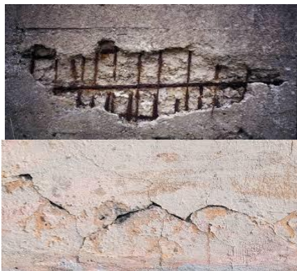
Fig. 1. Concrete spalling with exposed and corroded working reinforcement
